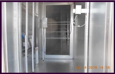
UV-C Lights Installed in HVAC Plenum
