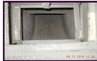
**Fire damper in open position before cleaning**
