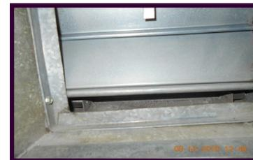
**Fire damper in closed position after cleaning**
